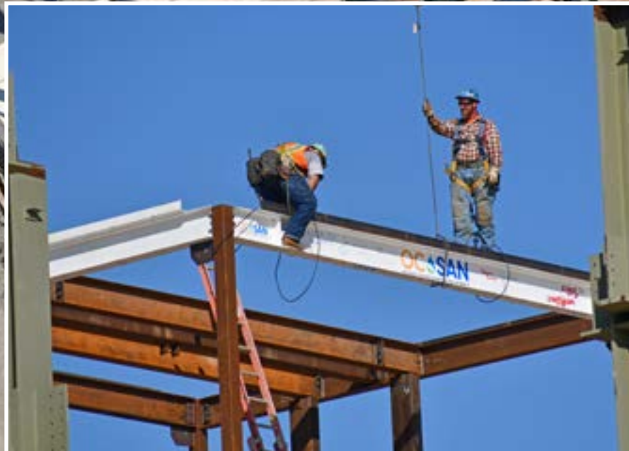
Construction of new OC San Headquarters in Fountain Valley.
